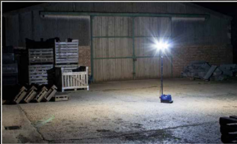
360° area flood lighting
